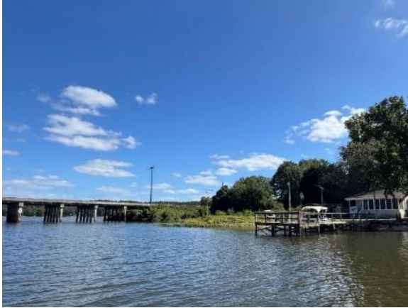
Proximity to Road Traffic
